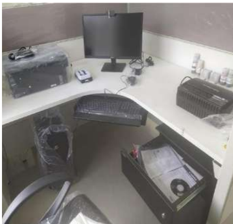
JORHAT DATA CENTER
