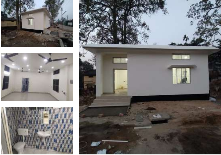
JORHAT - Civil construction data centres
